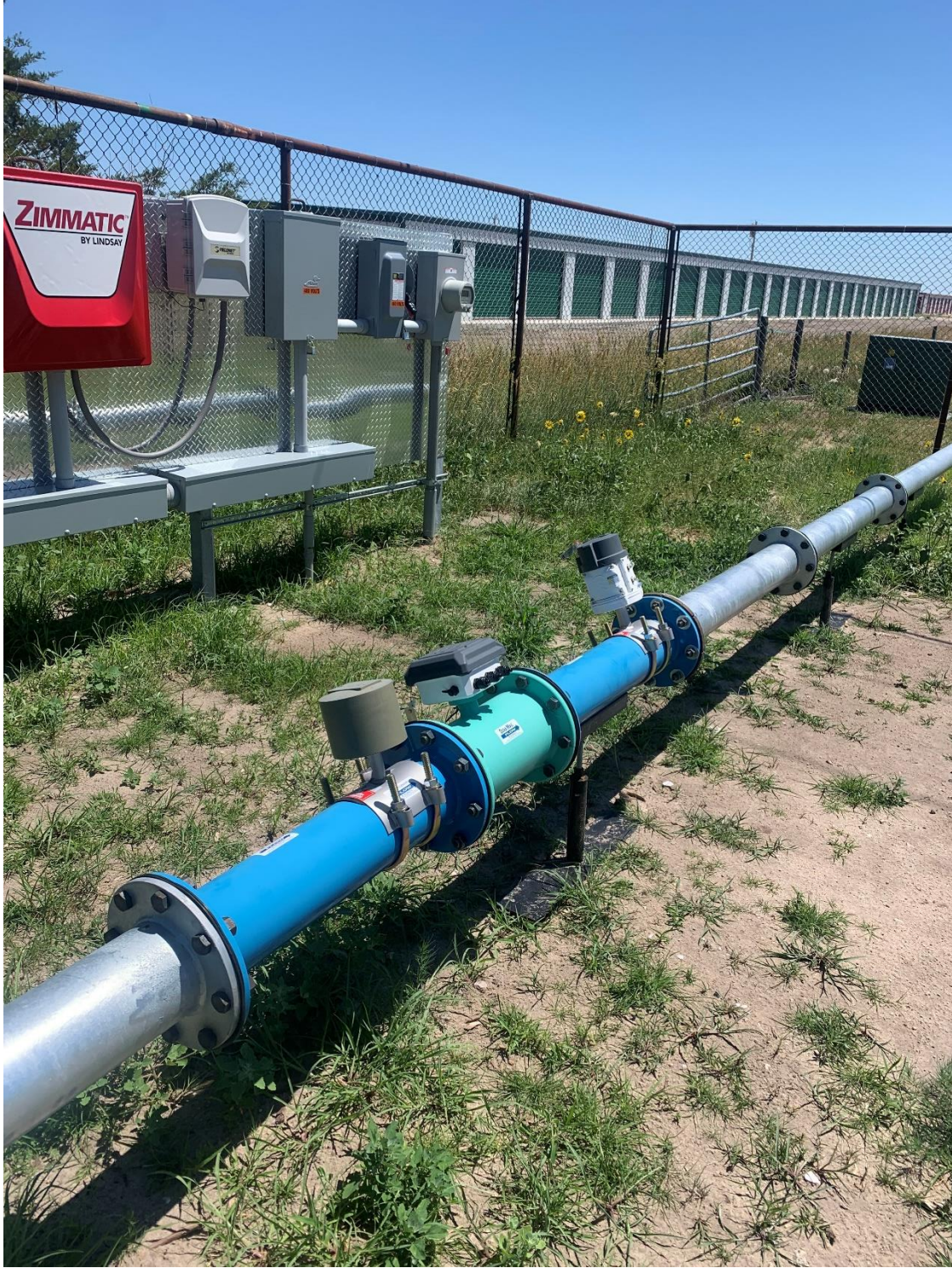
Multiple different types of flowmeters and a high tech panel board allows for many educational opportunities.
